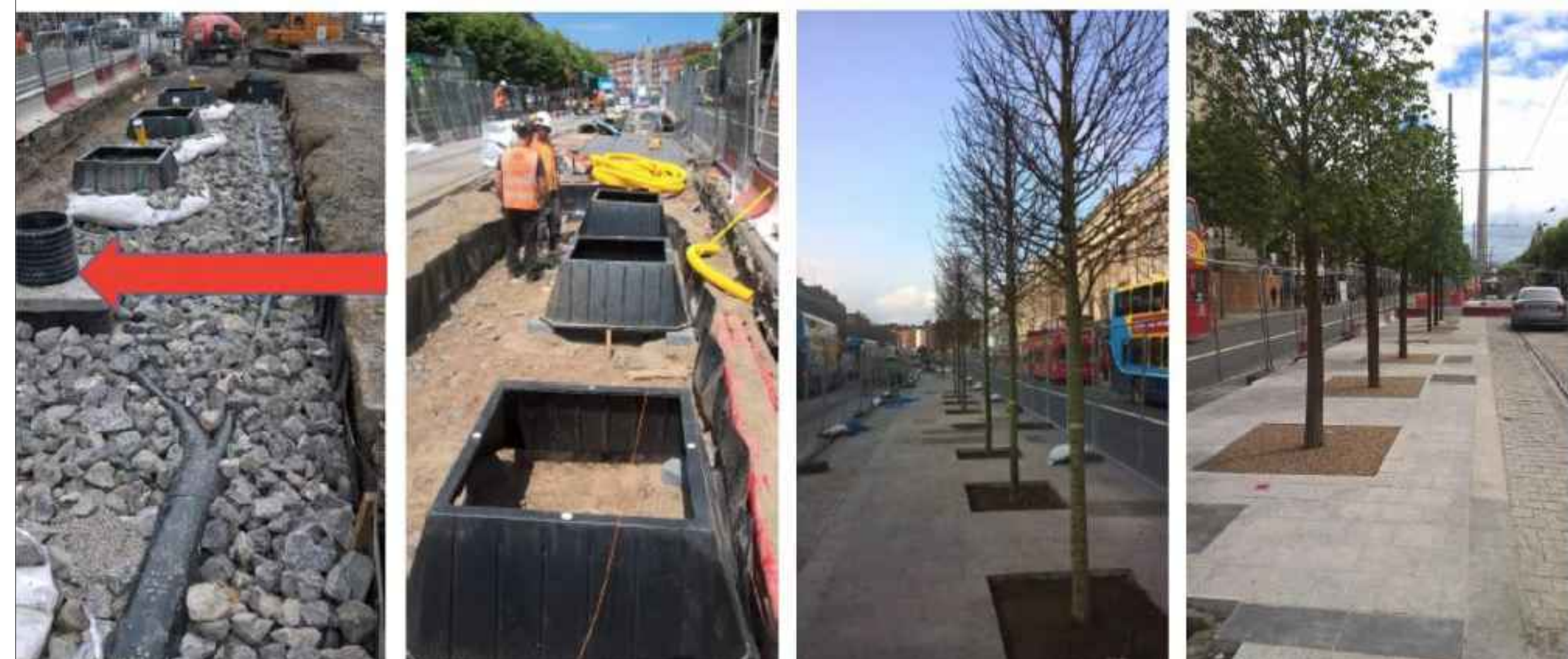
FIGURE 1: NATURE-BASED SOLUTIONS (NB SUDs): STOCKHOLM METHOD FOR PLANTED TREES
